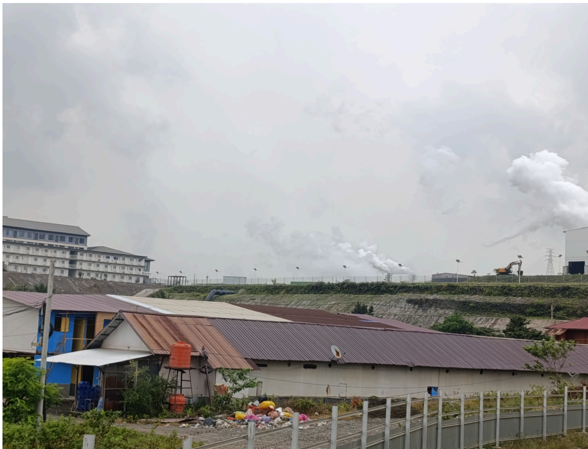
Figure 15 — Coal plant for nickel smelting, a joint venture of Jiangsu Delong Nickel Industry (currently in Administration), and Dexin Steel Indonesia (PTDSI), in Indonesia Morowali Industrial Park (IMIP); photo and text by Nursadah K, 6 October 2025
